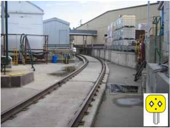
Restricted clearance in a customer siding Inset: Restricted clearance sign
